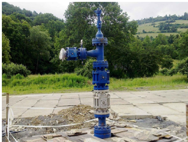
Fig. 13 New wellhead of the Poręba Wielka IG-1 well (photo: B. Bielec)
