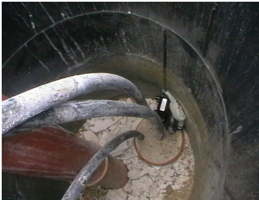
Fig. 22 Cerneves site July 2023. Top right: inlet to the technology (see Figs. 13, 14)
