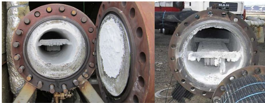
Fig. 4 Heavy silica scaling in the surface equipment of the IDDP-1 well during discharge testing (Karlsdottir et al. 2015)
