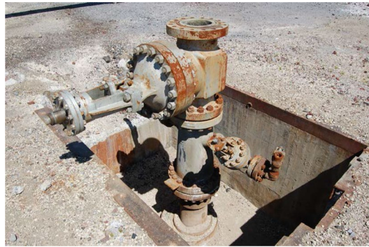
Fig. 5 The wellhead of the abandoned H-43 well in the Los Humeros geothermal field (photo: Michal Kruszewski)
