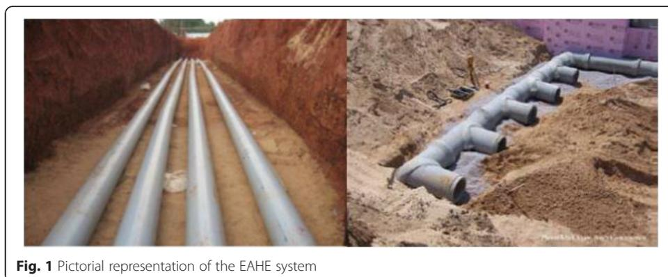
**Fig. 1** Pictorial representation of the EAHE system
